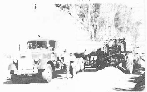
BIG OPERATION went on this week resurfacing oiled top on Tavern Road. Here Cynthia's photo shows tanker and spray truck putting oil onto sand that trucks spread ahead. See photos inside.
