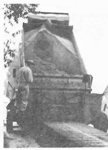
HERE truck tows trailer-spreader which lays sand in even row at side of road. Next page shows blade mixing oil and sand into finish mix which is then spreads smoothly, becomes fine new surface for increasing traffic.
